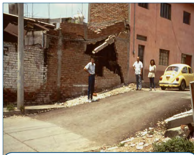
MAJOR LAND SUBSIDENCE IN RURAL MEXICAN TOWN RESULTING FROM EXCESSIVE WATERWELL ABSTRACTION
